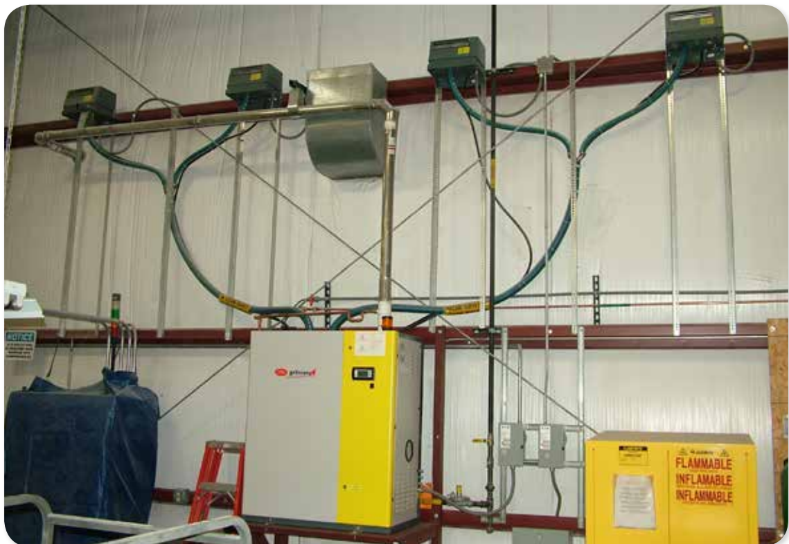
gaSteam with distribution directly into the environment
