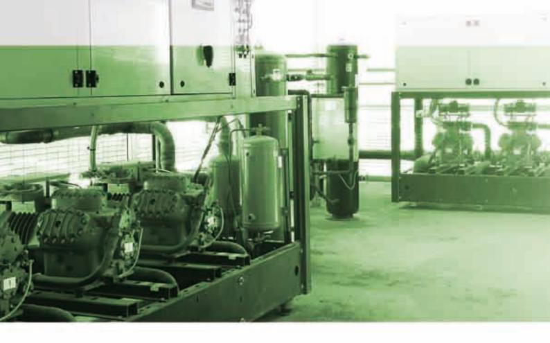
The compressor rack is the most important and complex electromechanical device in the refrigeration system: this delivers cooling for the foodstuffs to all the refrigeration utilities and the related processing rooms.
