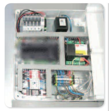
the electrical panel was fitted to manage the changeover in technology between PWM and E<sup>2</sup>V manually or via PlantVisorPRO
